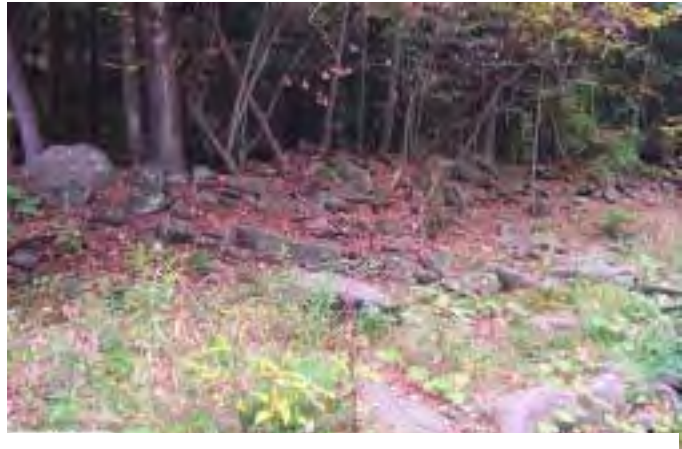
Photo 3. Cobble and earth berm, on right bank in the pond area. The main stream is behind the viewer, flow is from right to left.
