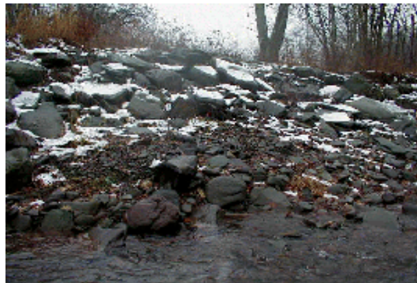
Photo 7. Boulder rip-rap, left bank, above private bridge at the top of MU8.
