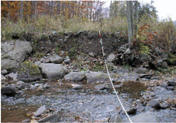
Photo 17. Eroding left bank at mowed field, monitoring cross-section 16, MU8.
