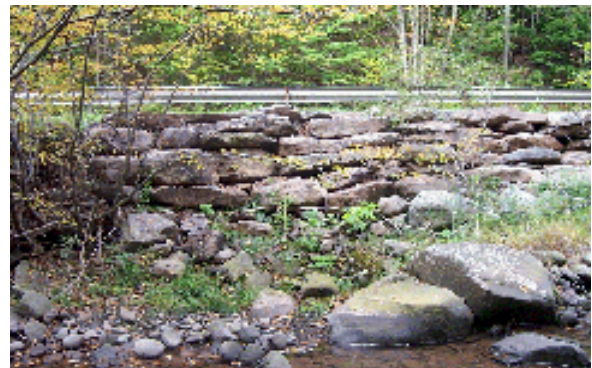
Photo 10. Stacked rock wall at monitoring cross section 15, MU8, 2002.
