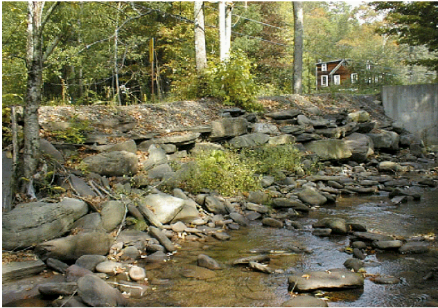
Photo 8. Stacked rock wall, right bank below bridge, MU8.
