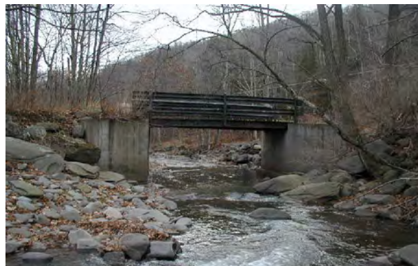
Photo 3. Private bridge near the top of the upstream section of MU8, looking downstream.
