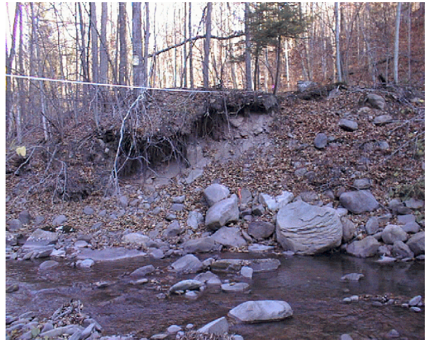
Photo 16. Eroding left bank at wooded area, at monitoring cross-section 14, MU 8.
