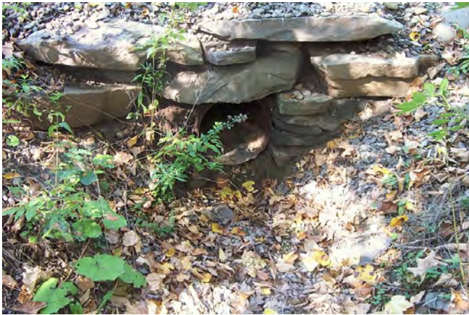
Photo 5. Middle culvert, right bank, MU8.
