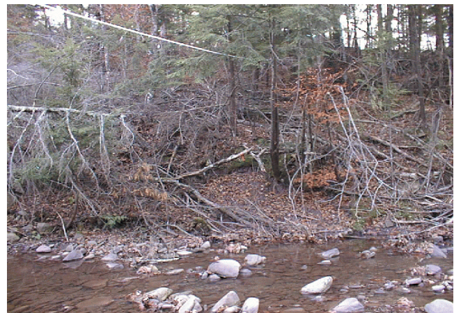
Photo 13. Eroding left bank at high terrace, monitoring cross-section 11, MU8.
