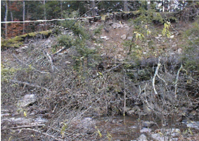
Photo 14. Eroding left bank at high terrace, monitoring cross-section 12, MU8.
