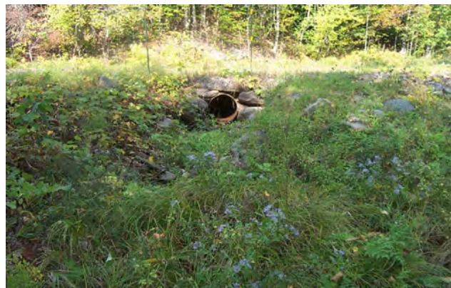
Photo 4. Upstream-most (top) culvert on the right bank, MU8.
