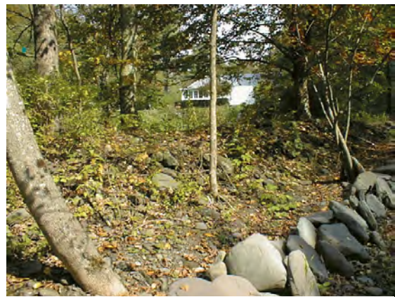
Photo 12. Earthen berm viewed from stream (at right), floodplain is on the other side, at left.
