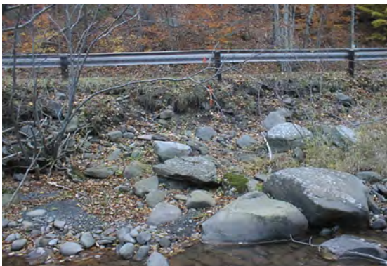
Photo 9. Eroding bank at monitoring cross-section 15, MU8, summer, 2001.
