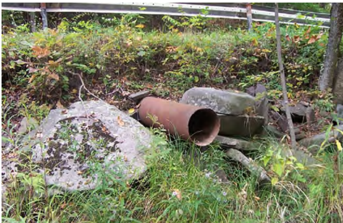
Photo 6. Bottom culvert, right bank, MU8.
