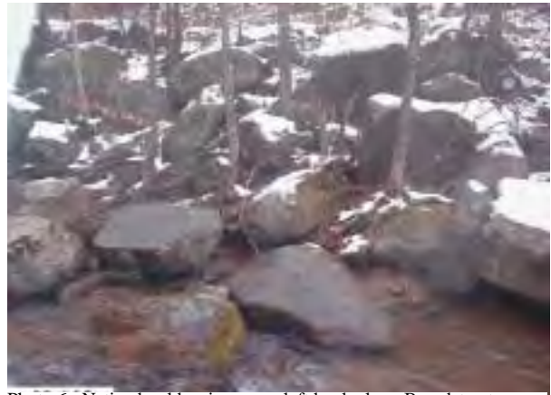
Photo 6. Native boulder rip-rap on left bank along Broadstreet Hollow Road, sparsely vegetated with trees. Flow in the stream is from left to right.
