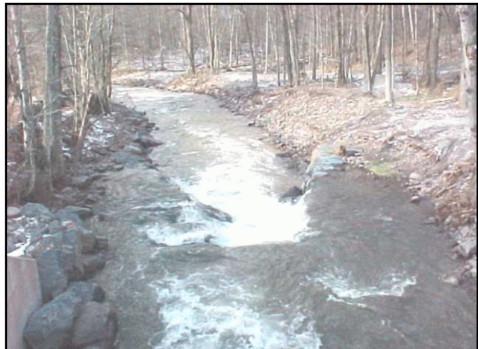
Figure III-24: View of a cross vane from upstream. Note that velocities are placed in the center of the stream channel and still, flat water is located along the banks upstream of the structure.
