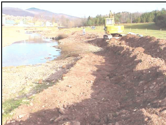
Figure III-25: Excavation of streambank benches and the placement of alternating lifts of soil and willow shoots is the basis of brush layering.
