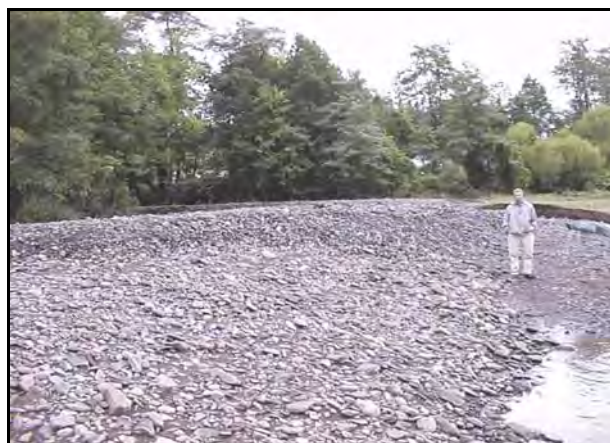
Figure III-11: Large gravel deposition, at the confluence of North Settlement Creek and the Batavia Kill, after Hurricane Floyd September 1999.
