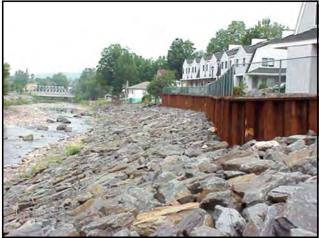
Figure III-21: Hardened streambanks can transfer erosional problems downstream.
