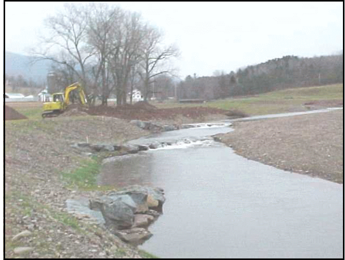
Figure III-23: View, looking upstream, of 3 rock vanes. Note that water is deflected away from the streambank.
