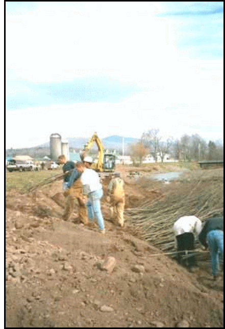
Figure III-26: Installing Brush Layering.
