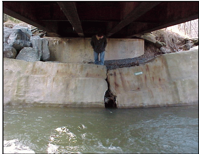
Figure III-18: Failure of bridge abutment due to localized degradation of the stream channel caused by inadequate bridge opening.
