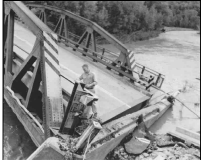
Figure IV-46: Bridges over the Batavia Kill or the tributaries have often been the subject of extensive damage due to flooding.
