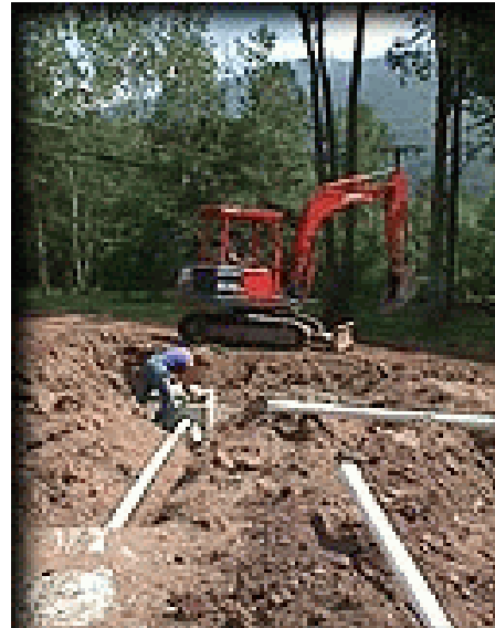
Figure IV-44: Replacement or upgrades of failing septic systems is a high priority of NYCDEP and the Catskill Watershed Corporation(CWC).
