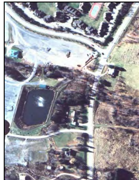
Figure IV-45: Aerial view of a stormwater treatment pond at Ski Windham. The pond captures runoff and provides a controlled release to the stream system.
