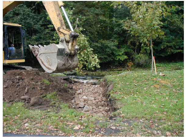
Photo 6. Swale expanded and filled with cobble; September 26, 2003.
