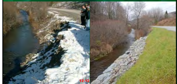
Town of Tompkins Readburn Road Site #2
