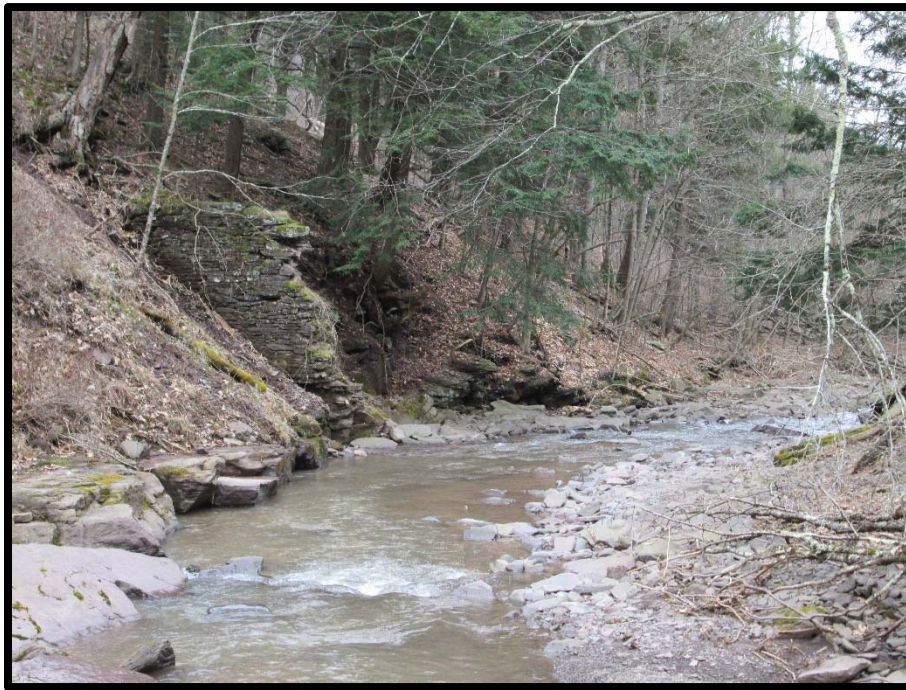
Figure 40: Photo Looking Downstream At Abandoned Dam
